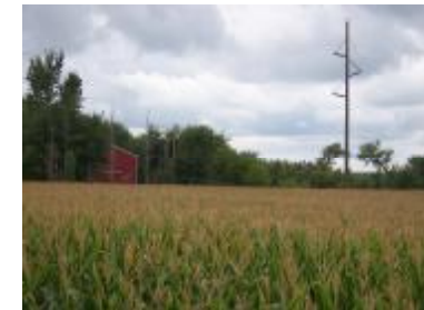
Above Ground Transmission Lines
