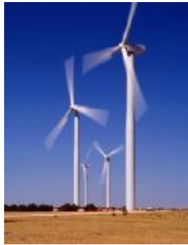
Tower (and access road)
